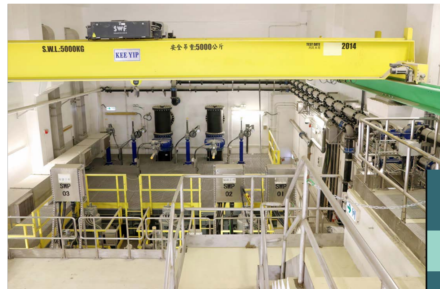
Bump engine of Happy Valley underground stormwater storage tank.
