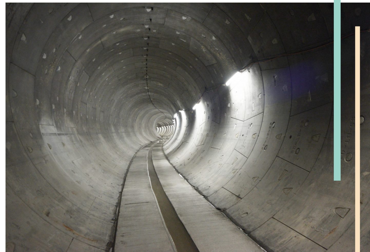
Lai Chi Kok Drainage Tunnel. Source: The Drainage Services Department.
